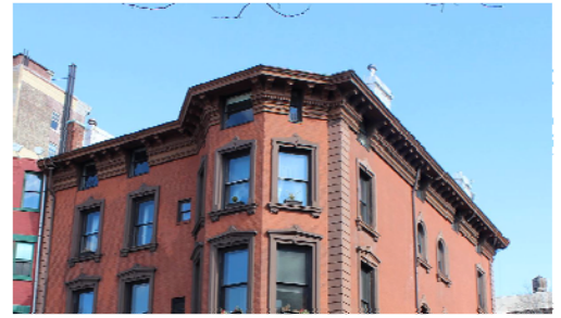
An older townhouse with a large cornice. Aside from being ornamental the cornice helps to keep the rain off the window heads and lets any run off drip to the grade and not get on the facade
