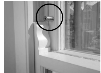
Figure 4. Sash stop. This will stop the window from opening more than a few inches
