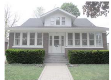
Figure 23. Hedges prevent access to any of the windows from the outside
